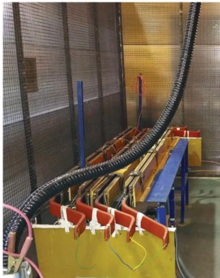
Generator Wound Bars and Coils Lab
